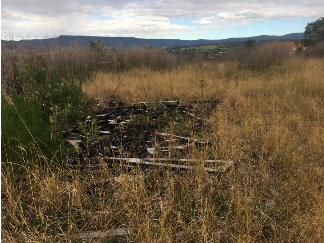
Photo 3: Burnt pile of building rubble south-west of the dwelling (22 July 2019)
