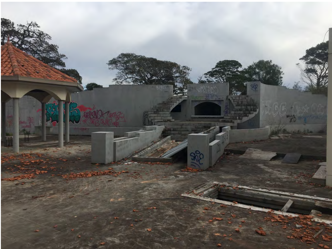
Photo 11: Northern view of carpark/basement, north of the dwelling (22 July 2019)
