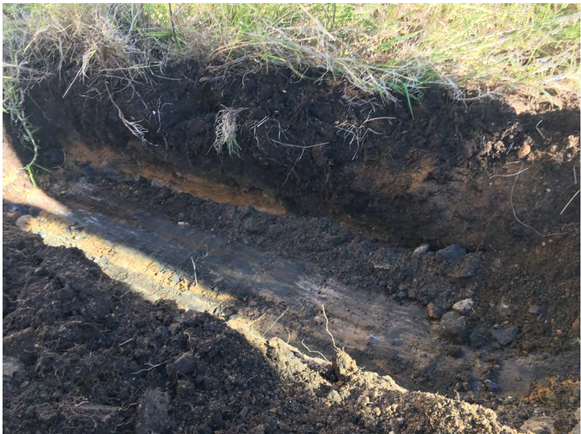
Photo 15: Test pit TP101 (24 July 2019)
