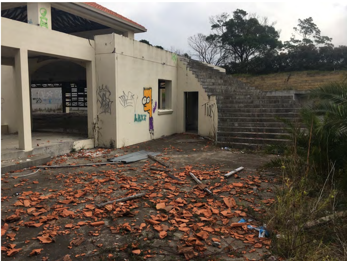
Photo 9: North-eastern side of the dwelling (22 July 2019)
