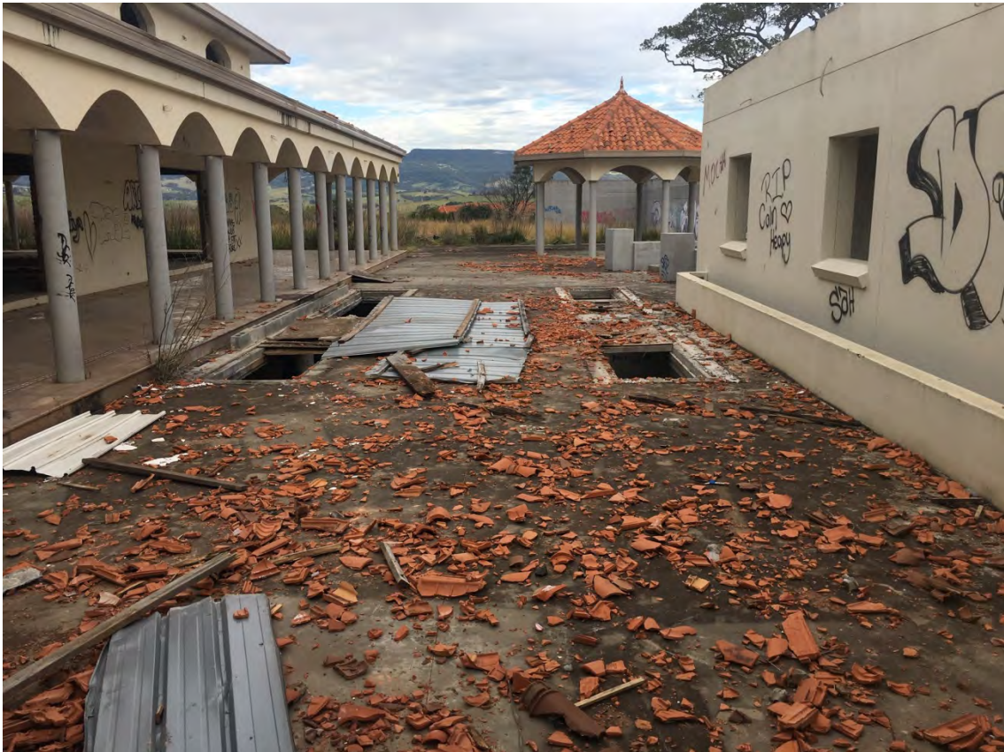
Photo 10: Western view in between dwelling and garage (22 July 2019)
