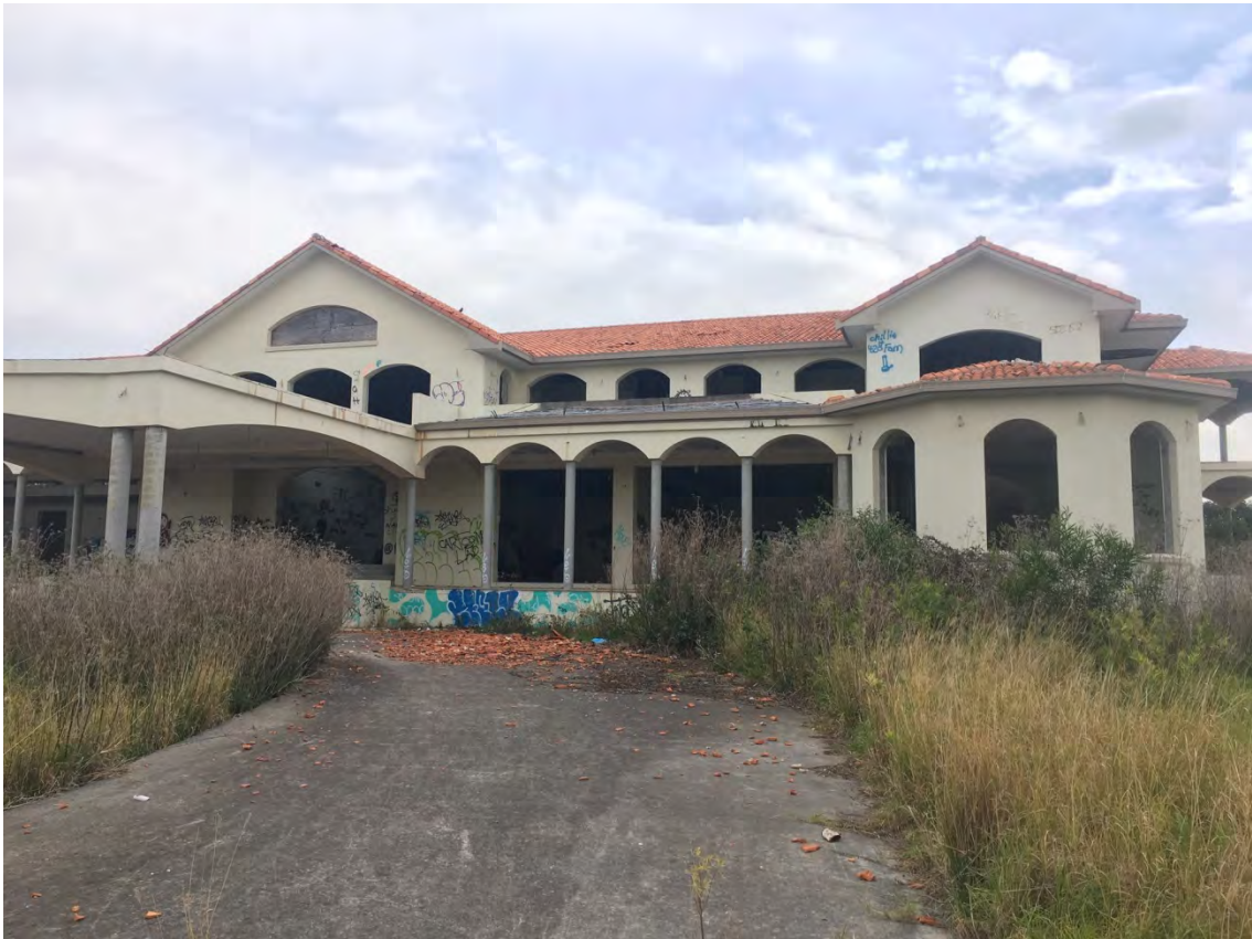
Photo 5: Northern view of the dwelling (22 July 2019)
