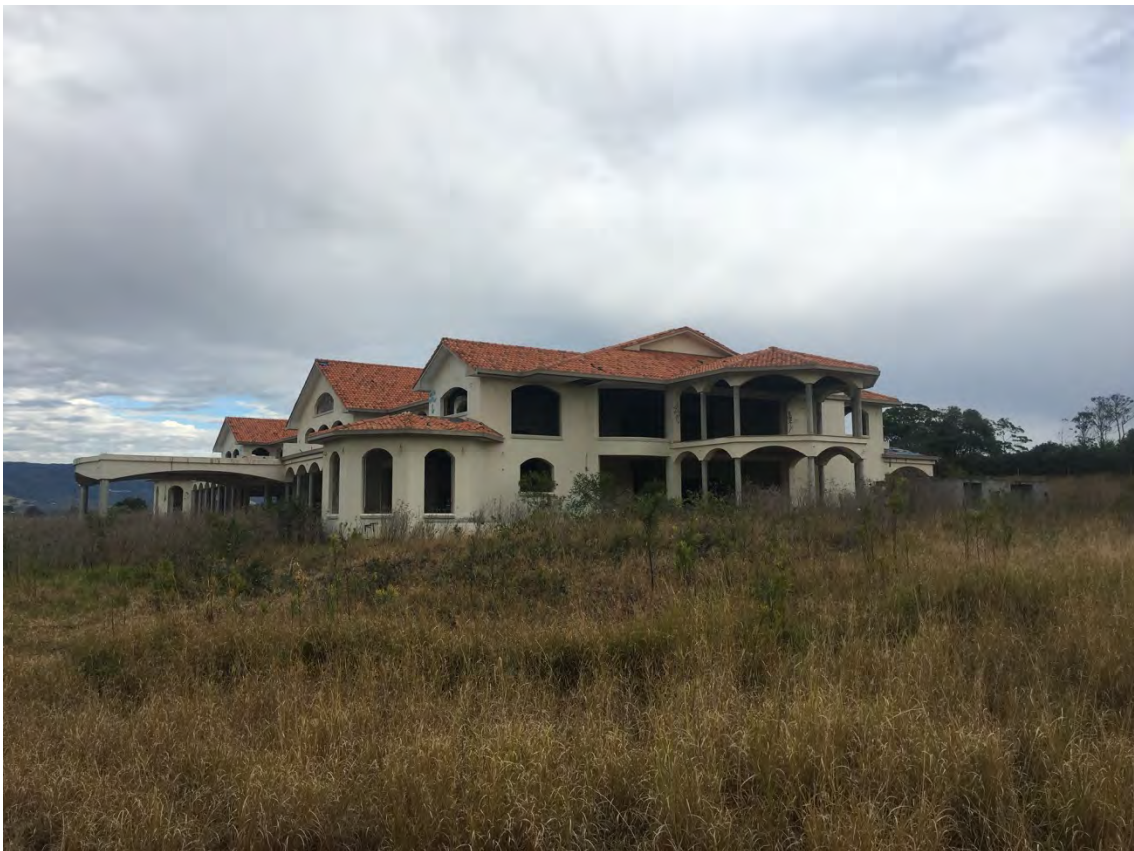
Photo 6: North-west view of the dwelling and surrounding vegetation (22 July 2019)
