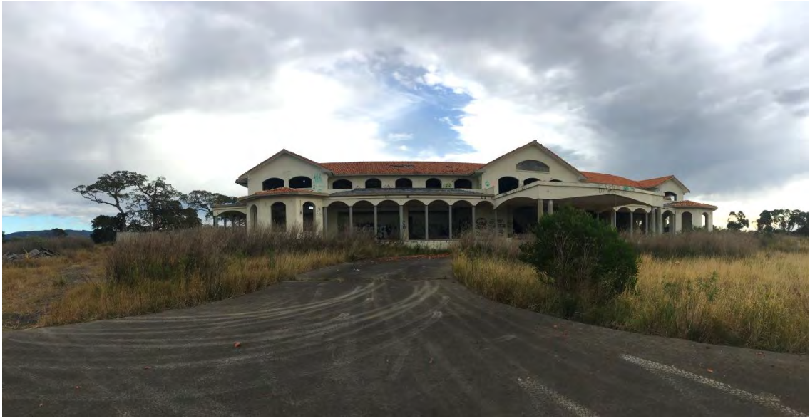
Photo 12: Northern view of the dwelling (22 July 2019)
